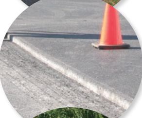
Paving notches are milled into existing asphalt and sealed to create a smooth transition and to prevent the new asphalt from getting thin.
