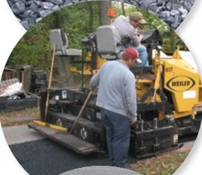
One of our primary objectives is to install a minimum of 1% slope to prevent puddles and promote proper water drainage.
